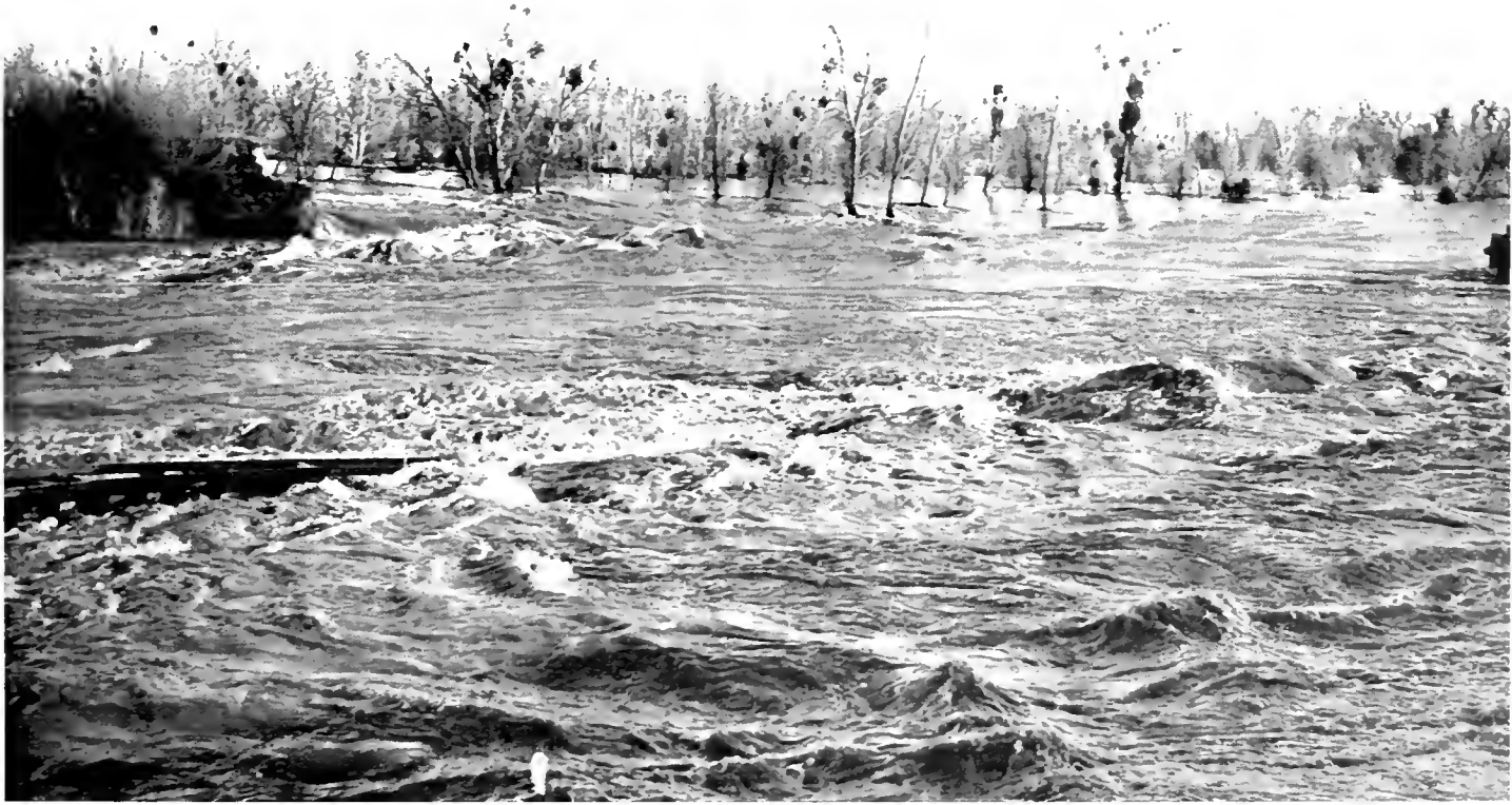
Break in Feather River levee of Reclamation District 803, Sutter County, that flooded 32,000 acres of farm lands
